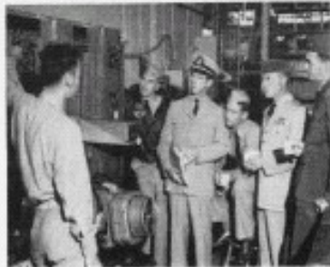
CHECK-OUT ON CAMERA CONTROLS SYSTEM
